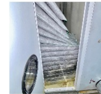
Figure C. Typical installation of secondary stage filter "pocket type" in an air handling unit
