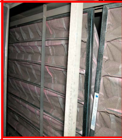
Correct and incorrect positions of the installation frame clip
